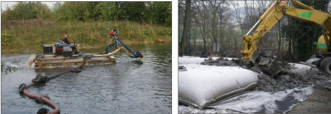
Abb. 3: Geotubes (<http://www.aquamarine-technologies.ch/geotube.html>)
